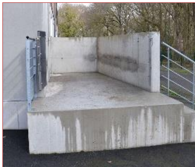
Figure 3.4 Solid concrete loading quay on farm that can facilitate loading operations.
