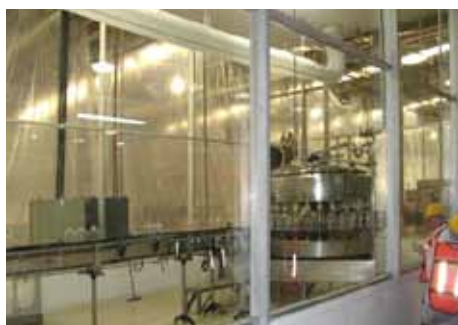
Screening to protect a filling zone during repairs
