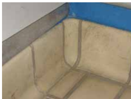
Detail of a hygienic floor with coved corners
