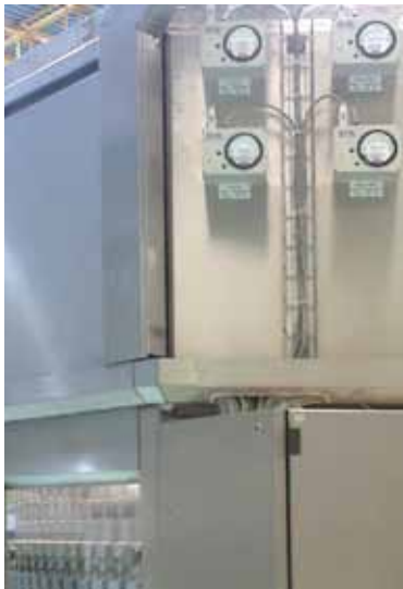
Pressure measurement of a filling cabinet
